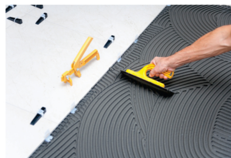
Stap4 : Apply adhesive & fix tiles
